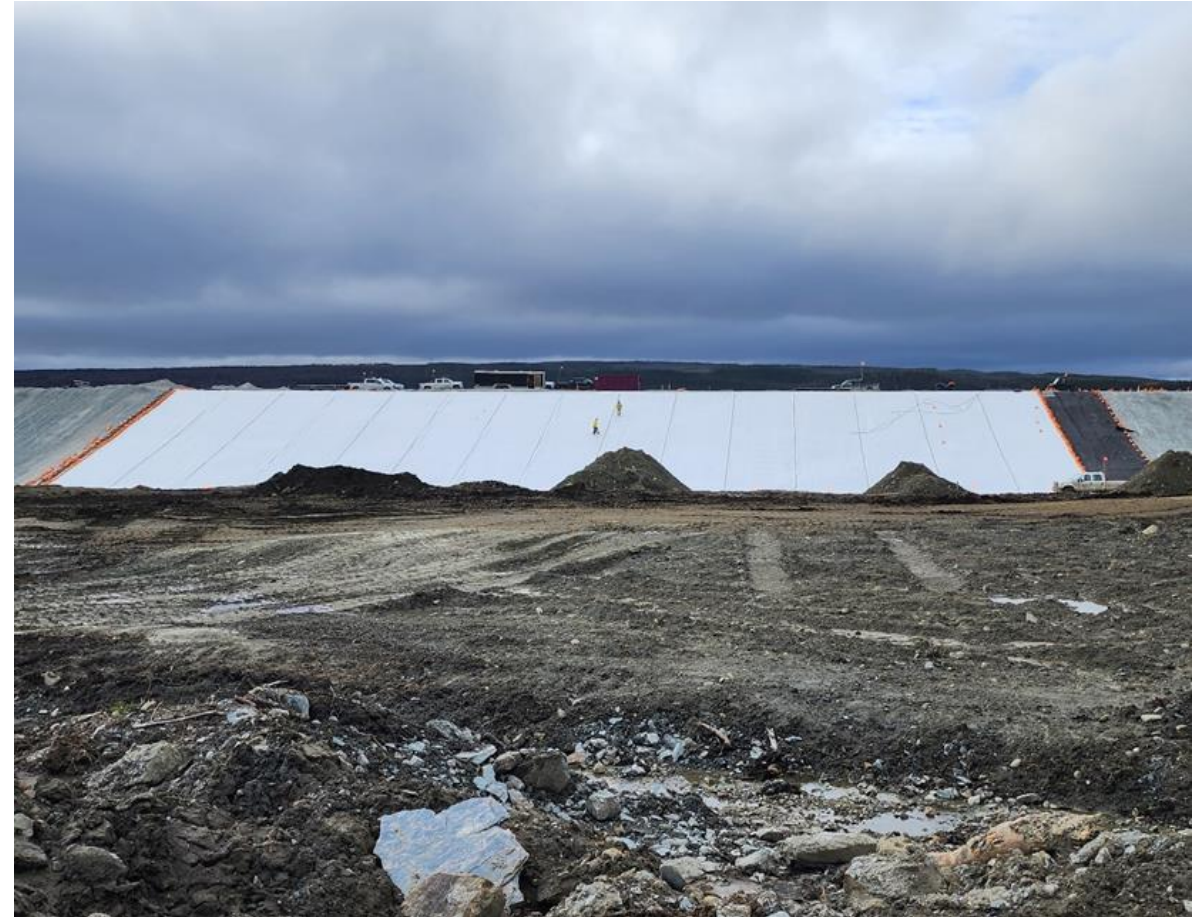
Tail Management Facility Liner Placement
