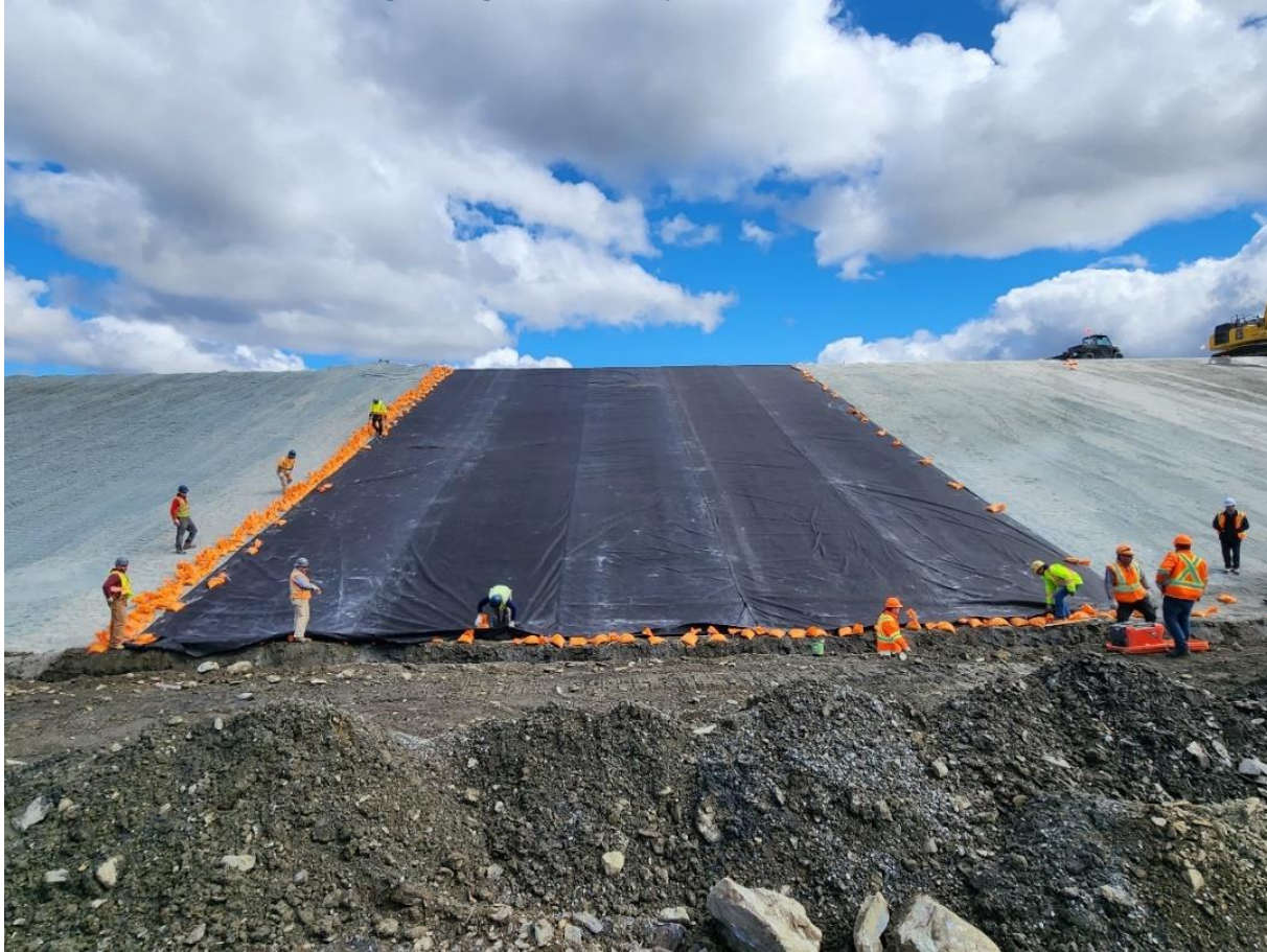
Tailing Management Facility Geotextile Placement
