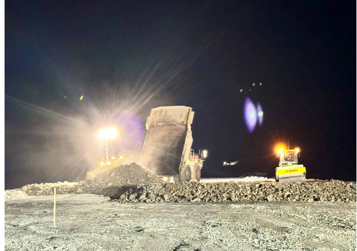
Tailing Management Facility Rock Placement
