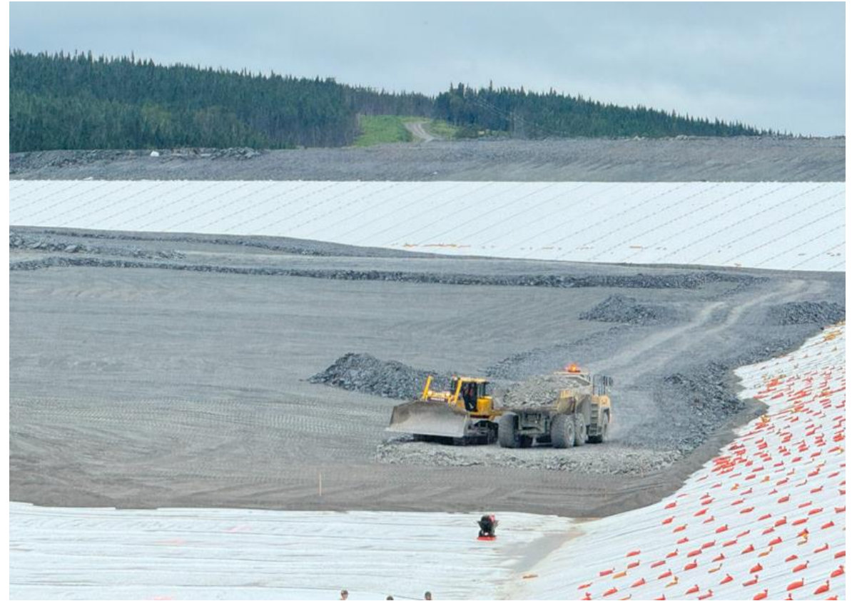
Tailings Management Facility Liner Progress
