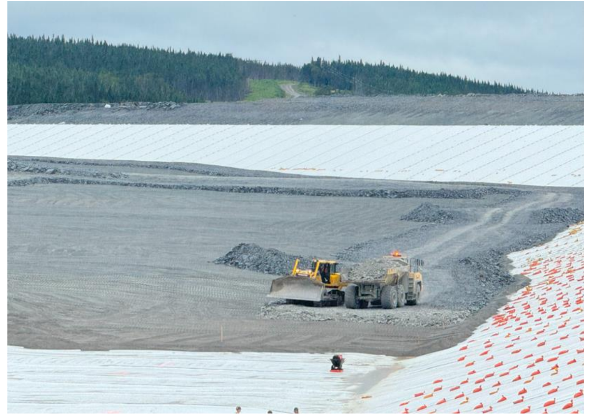
Tailings Management Facility Liner Progress
