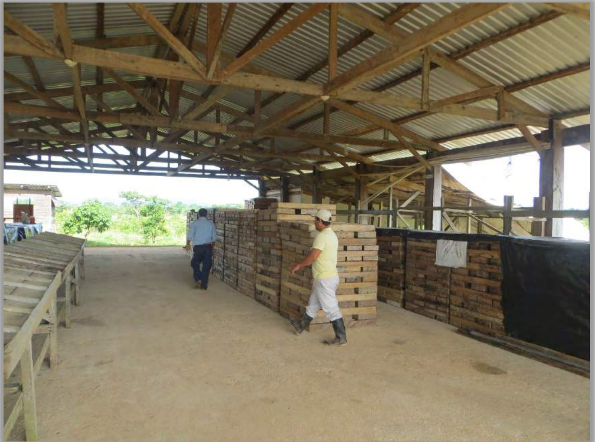
Figure 10.6 Core Storage Facility
