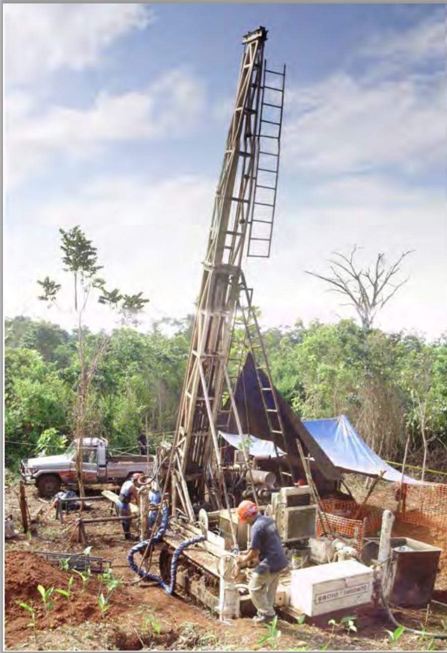
Figure 10.1 Rodio Swissboring Diamond Drill Rig
