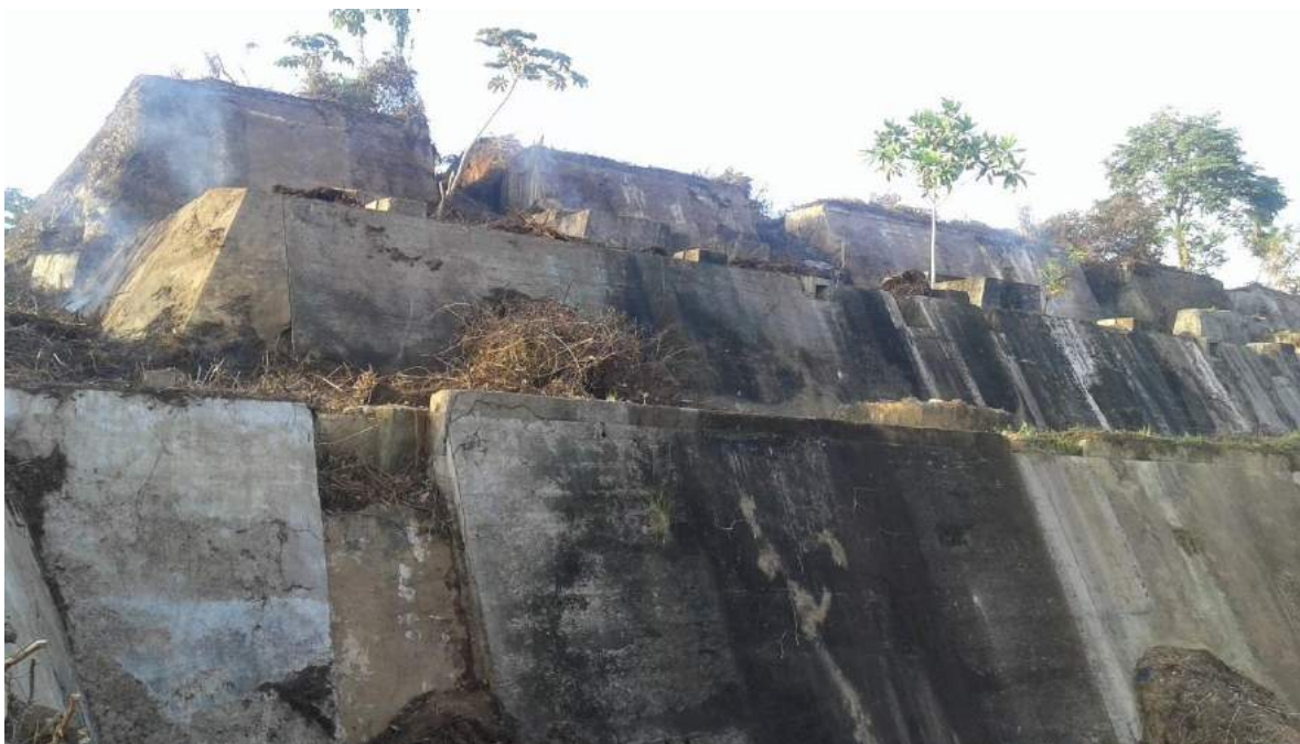
Photo 17.2 Photograph of existing old plant area – after clean-up (DENM 2016)
