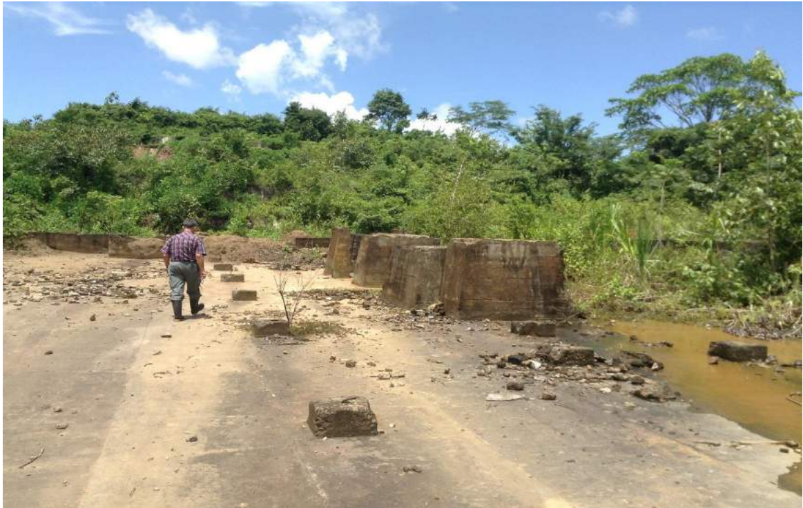
Photo 17.1 Photograph of existing old plant area – Mill slab area (DENM 2016)
